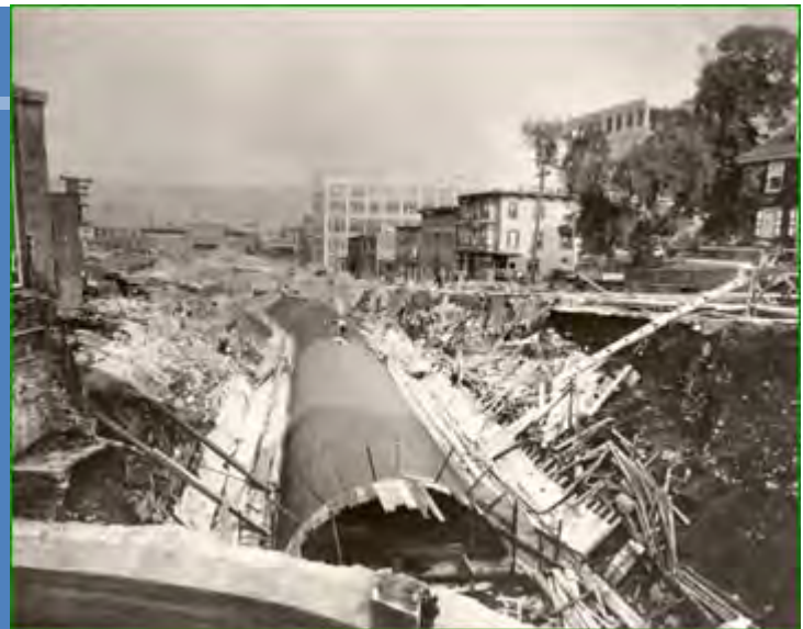
Flume construction to cover the final 2000 feet of the Saw Mill. Source: PS&S Integrated Services— http://www.psands.com
